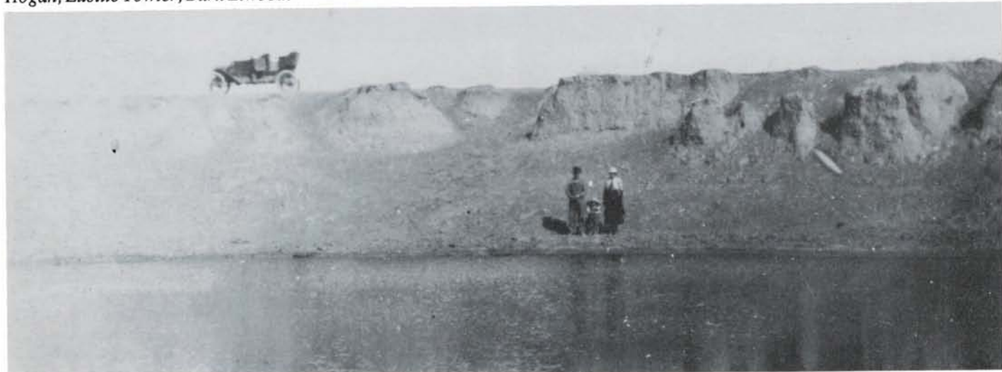
DEVIL'S HOLE, located in the northwest part of Grant County, was thought to be caused by the underflow of Bear Creek. In the early 1900's the hole was several rods across, had steep banks and was 35 to 40 feet deep.
