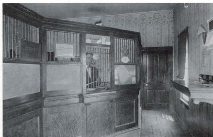
GRANT COUNTY STATE BANK, 1912. Lewis Wilson, Cashier at window.
