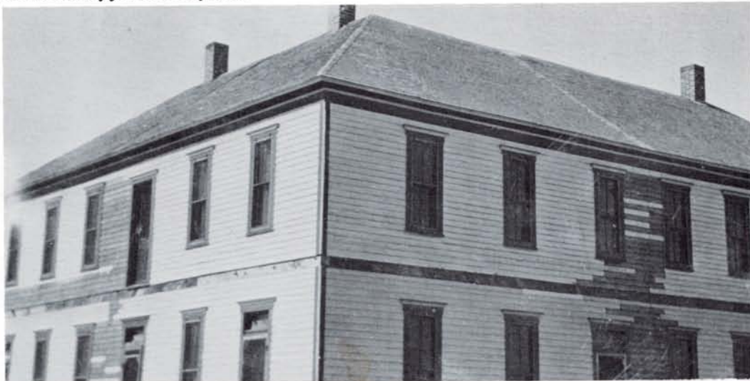
HOTEL after it was patched together, and before the porch and balcony were put on.
