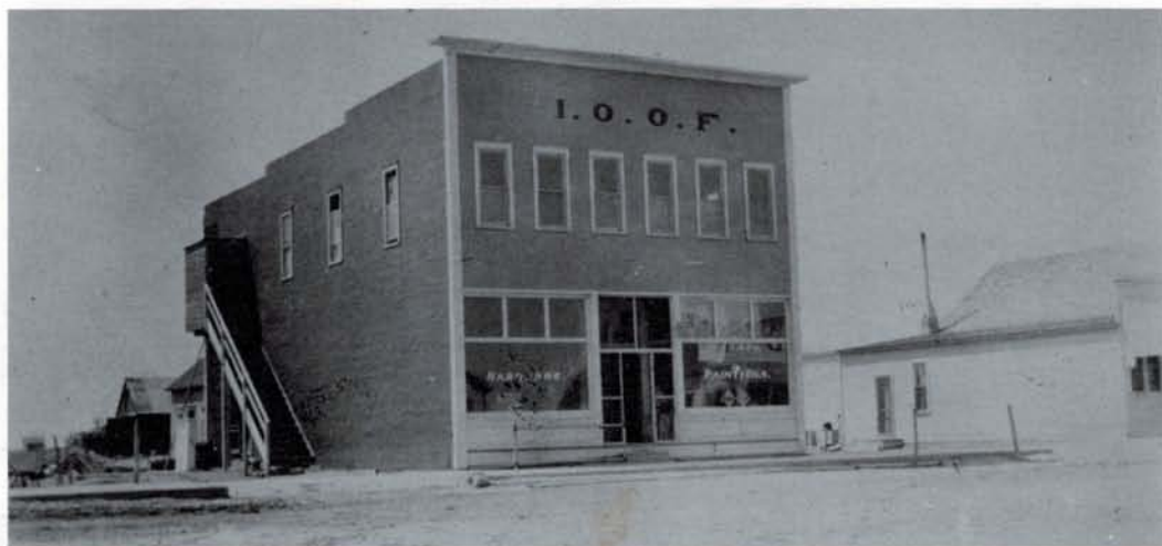
HIATT GENERAL STORE and meeting hall was the second new business to be constructed in the new town. The store was on the ground floor and the large room above was used for many community functions, dances, lodge meetings, oyster suppers, and it was even a skating rink offering feather pillows for rent with the skates.
