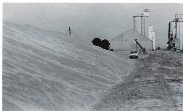
WHEAT PILED ON THE GROUND AT MILEPOST.
