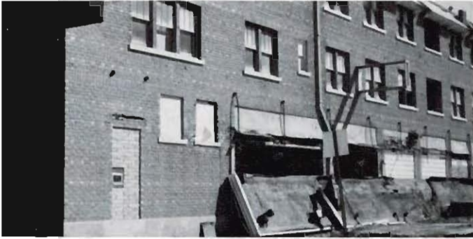
SPRING OF 1989, demolition of the Ralsamore Hotel.
