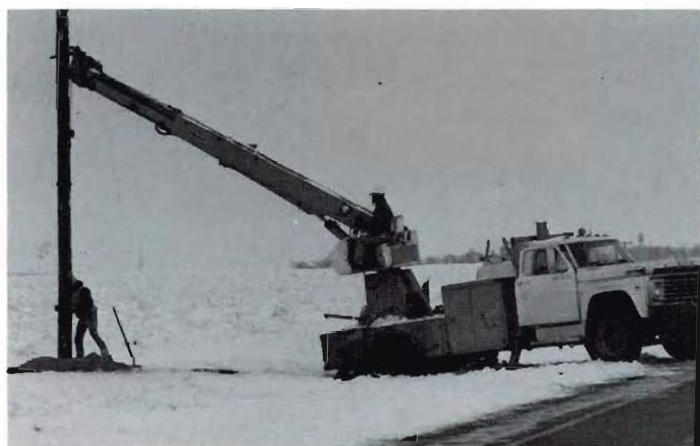
WINTER OF '77. Pioneer Electric repairs lines that have been downed by the ice storm.
