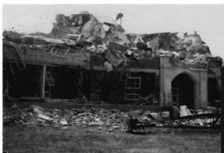
1973 DEMOLITION of the original high school building.
