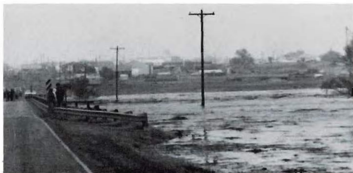
1976, NORTH FORK flooding south of Ulysses.
