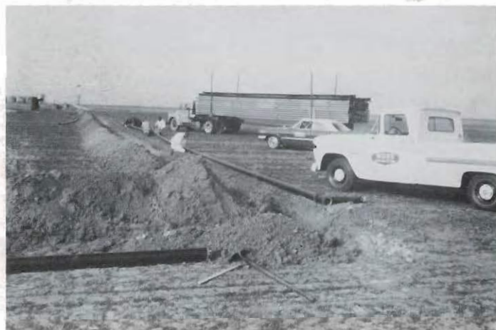
WORKERS FROM ULYSSES IRRIGATION PIPE COMPANY install an underground line, October, 1964.
