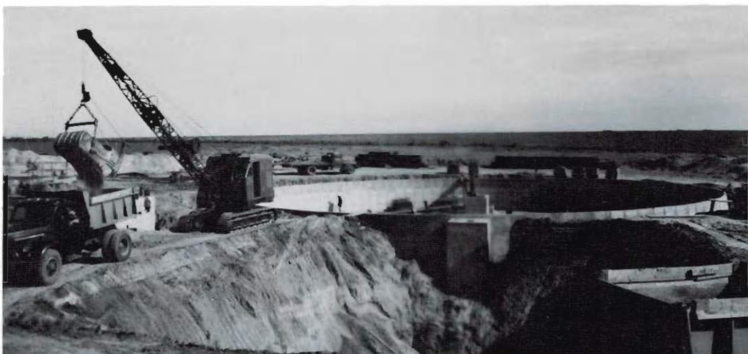
CITIES SERVICE HELIX PLANT under construction.
