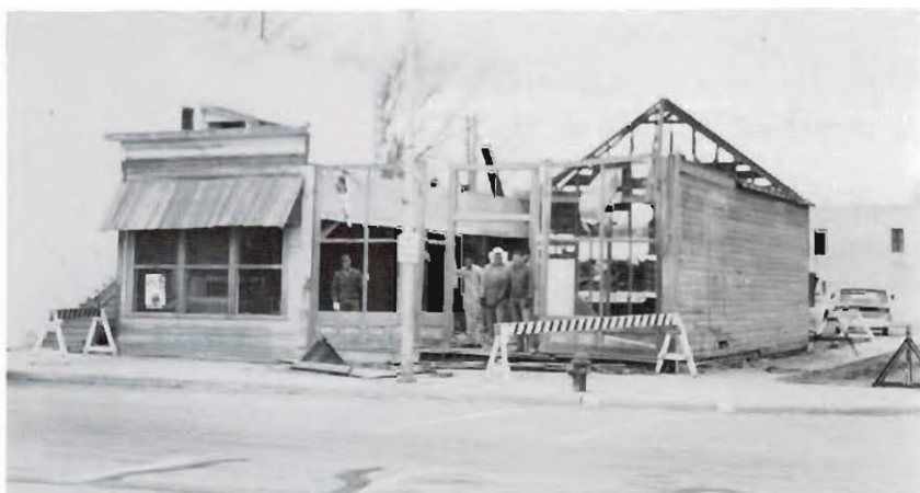
DOWN COMES THE OLD, tearing down Charlie Binney's Grocery Store.
