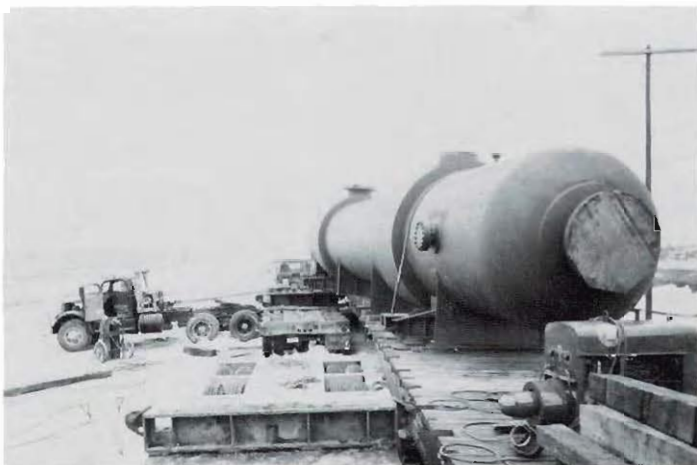
CONSTRUCTION WORK at the site of the new Cities Service Helix Plant, 1965.
