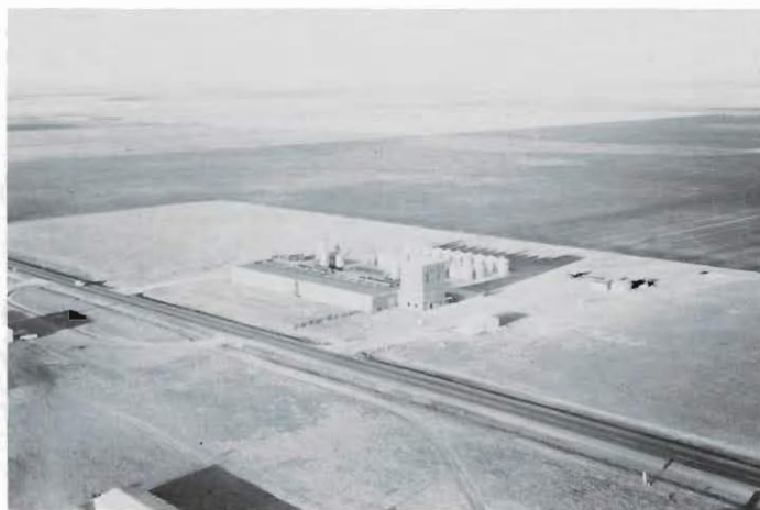
AERIAL VIEW of the Dekalb Agriculture plant, March 1961.
