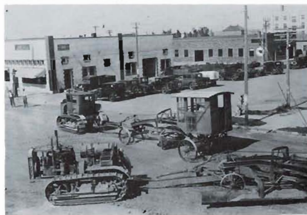
1930'S SOUTH MAIN, with equipment ready to begin street improvements.
