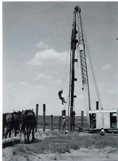
PILE DRIVER on the Cimarron River Bridge, 1935.
