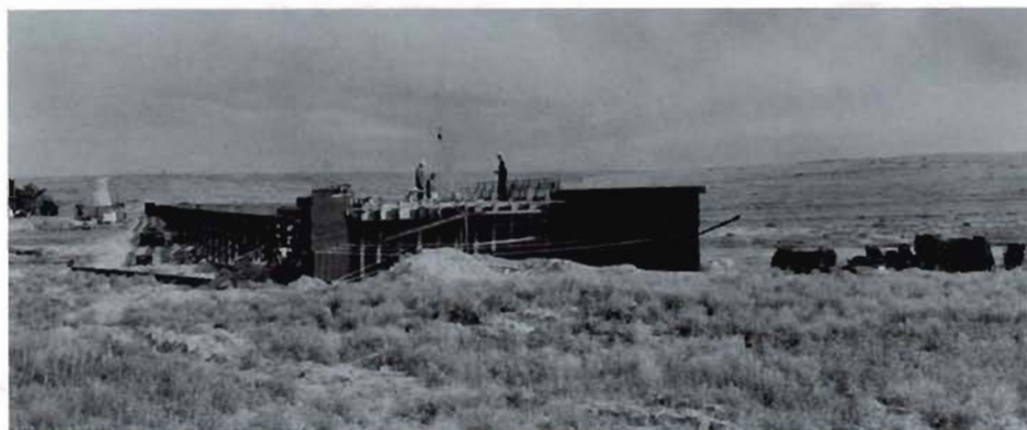
SPRING 1935, construction on the (early) Cimarron River Bridge.
