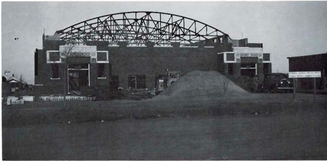
HIGH SCHOOL GYM UNDER CONSTRUCTION, built with W. P. A. funds.
