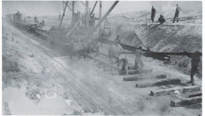
LAYING RAIL at present site of railroad bridge, 1922.
