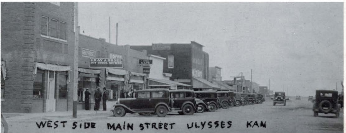
MAIN STREET, 1929. Construction on the Hotel Ralsamore has begun. The Hickok Building on the left is new.
