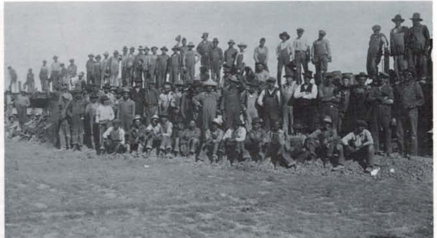
RAILROAD CREW, with the work train in Ulysses.
