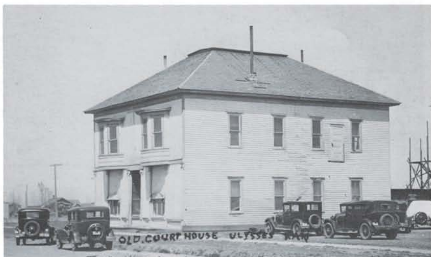
OLD COURTHOUSE, ULYSSES. Construction of the new courthouse can be seen in the background.
