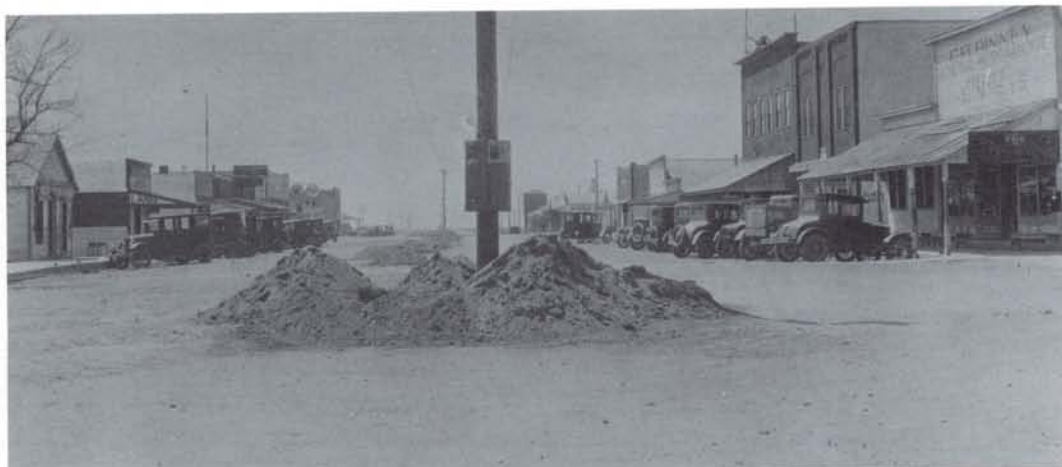
ELECTRICITY comes to Main St., 1925.
