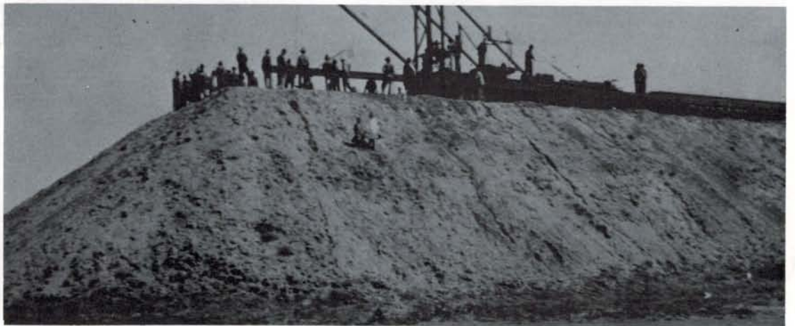
PILE DRIVER east of town at the site of what is now the Railroad Bridge, 1922.
